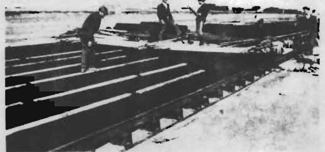
Fig. 3—Placing of paper; to protect the paper against wind, it is loaded with wood lathes
