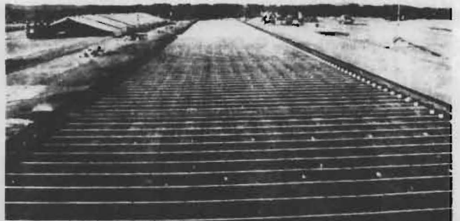
Fig. 6—Prestressing arrangement prior to concreting (note protective tents at left)
