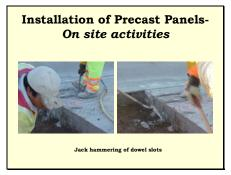
The dowel slot cutting and preparation includes (i) initial grooving to the required depth with a concrete saw; (ii) jack hammering of the concrete to carve out the dowel slot.
