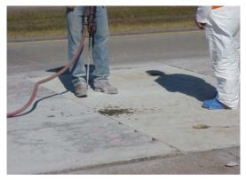
c) Drilling of injection portholes.
