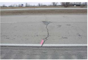
a) Deteriorated joint with cold patch with spalling.
