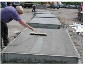
b) Concrete placement for precast panels.
