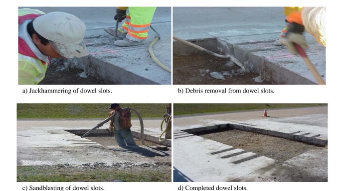
Figure 6. Preparation of the load transfer slots.
