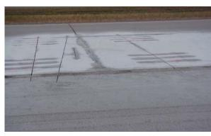
b) The existing slab after sawcutting.
