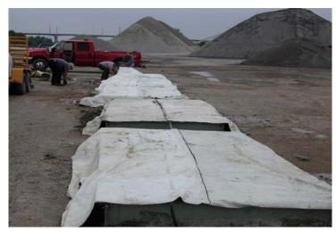
d) Curing of precast slabs.
