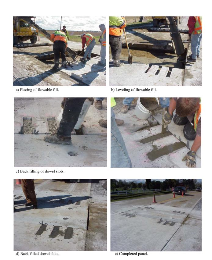
Figure 9. Flowable fill operation and dowel slot backfilling.
