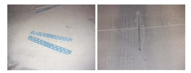
Figure 25. Fiberglass stitches.
