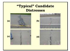
Typical distresses include (a) deteriorated joints with asphalt cold patch (b) medium severity mid panel cracking with associated spalling, (c) high severity transverse cracking, and (d) deteriorated joint (sealant damage) with associated spalling.
