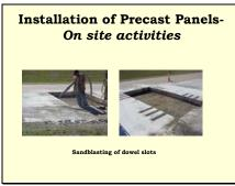
The dowel slot preparation also includes (i) air cleaning of dowel slot to remove debris and any loose concrete pieces; and (ii) sand blasting of the dowel slots. The dowel slots are approximately 4" wide and 5.25" deep (base of the slot cut).
