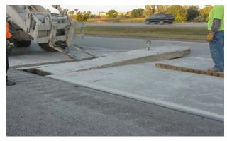
c) Removing the existing slab.
