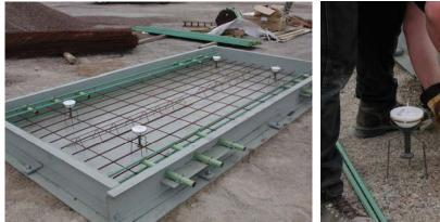
a) Reinforcement and dowel bar placement in the formwork.
