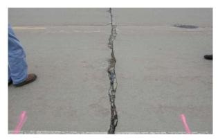
c) High-severity transverse crack.
