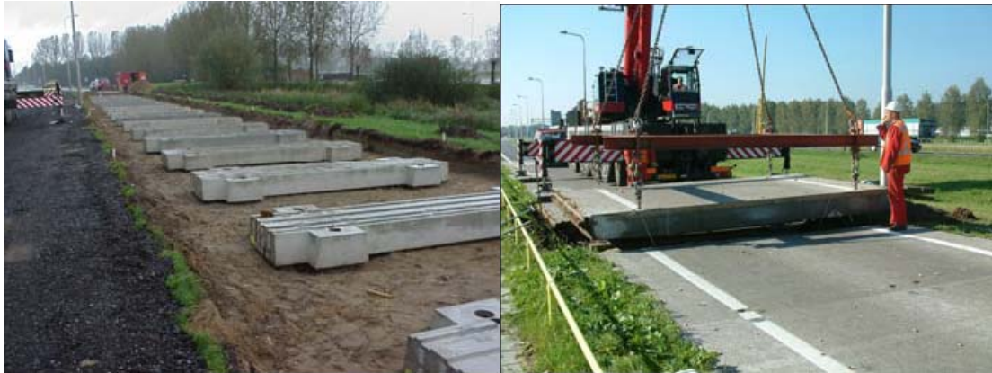
Figure 1. The ModieSlab test section along motorway A50.
