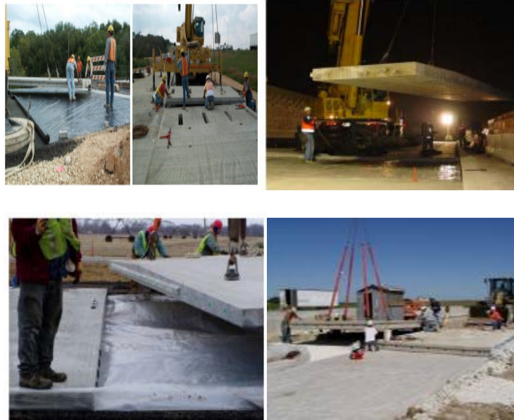
Figure 5. Precast slab projects in Texas, California, Missouri, and Iowa sponsored by the Federal Highway Administration (1).
