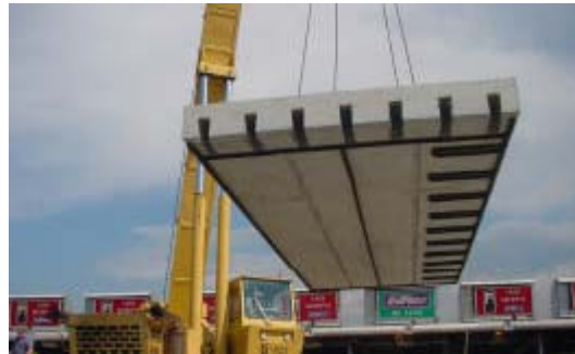
Figure 9. Bedding grout channels and gaskets.
