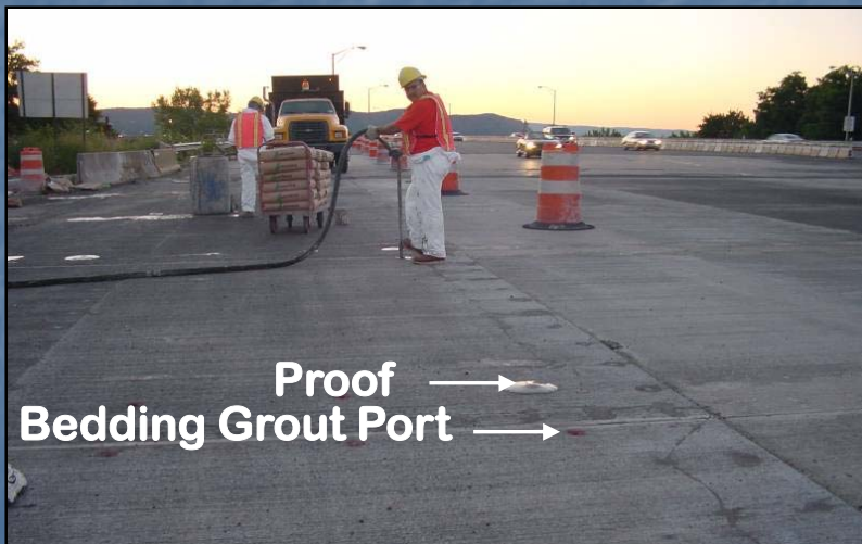
Pumping Bedding Grout
