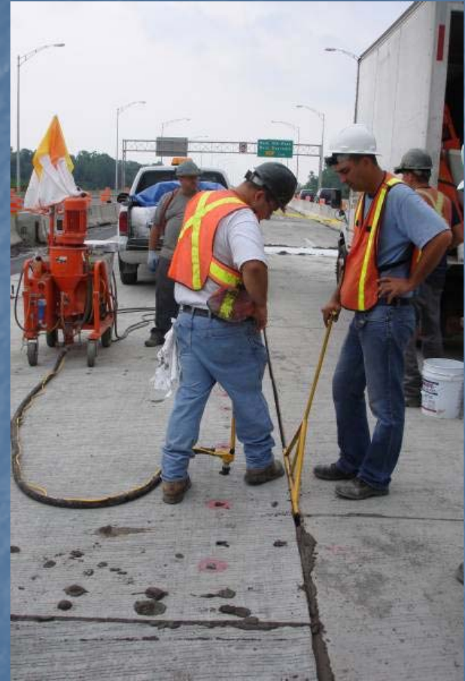
Contractor-Designed Joint Dam (Montreal Project)
