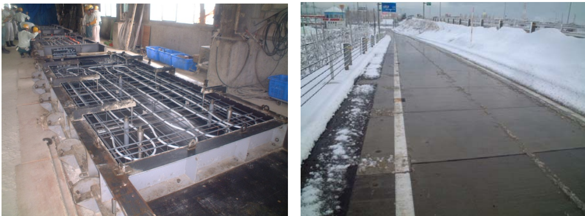
Figure 16. Heated precast panel fabrication and installed project
