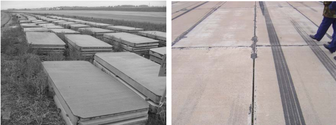
Figure 22. Soviet era precast panels – storage and installed site
