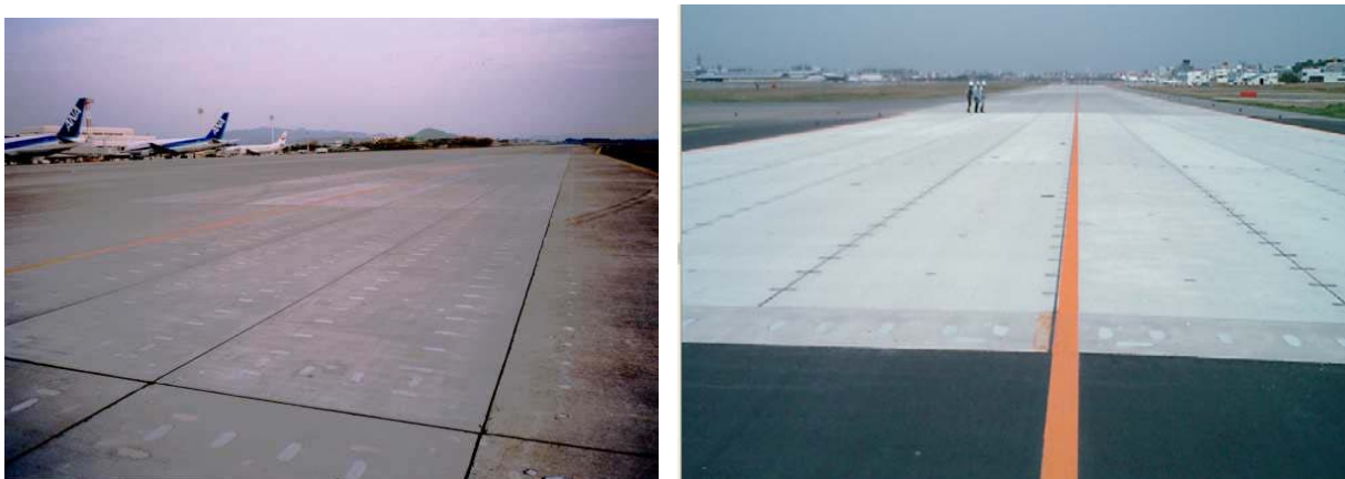
Figure 11. Airport applications (Osaka airport, 1998; Fukuoka airport, 2003)
