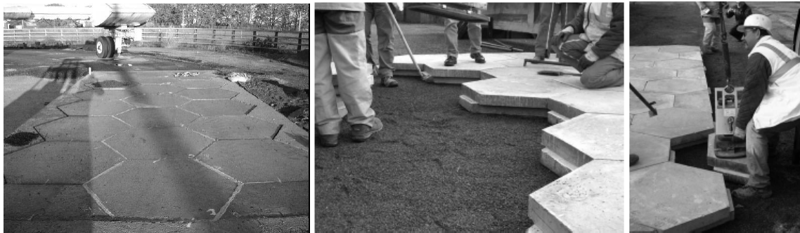
Figure 1. Installation of keyed hexagonal slabs
