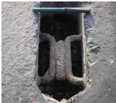
Figure 23. Welded lift loop connection
