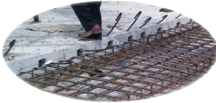
Figure 7. Use of cast-in-place reinforced end slabs
