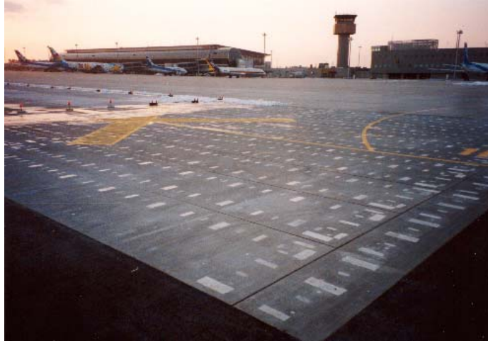
Figure 14. Constructed PCP at Sendai Airport
