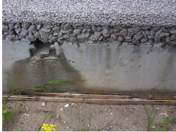
Figure 18. The two-layer porous surface
