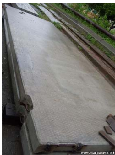
Figure 21. Russian standard design precast panel
