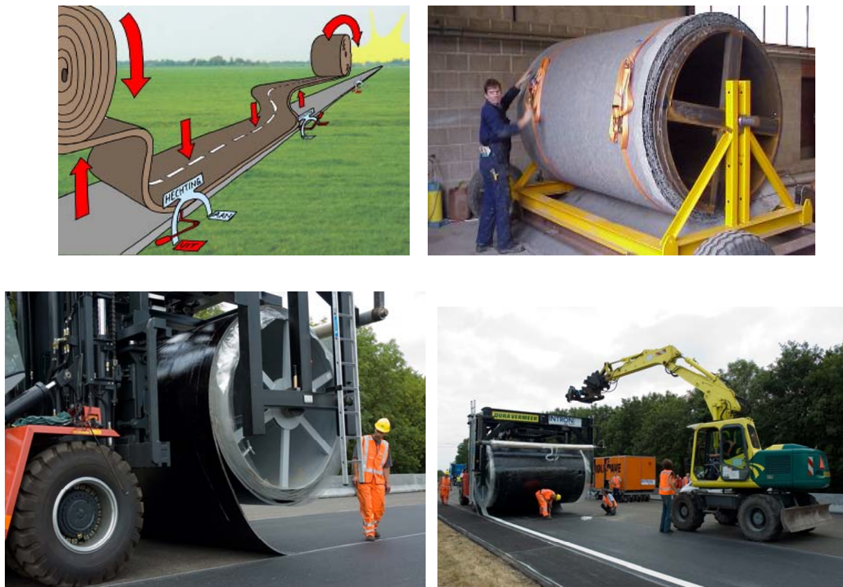
Figure 20. RollPave features and installation
