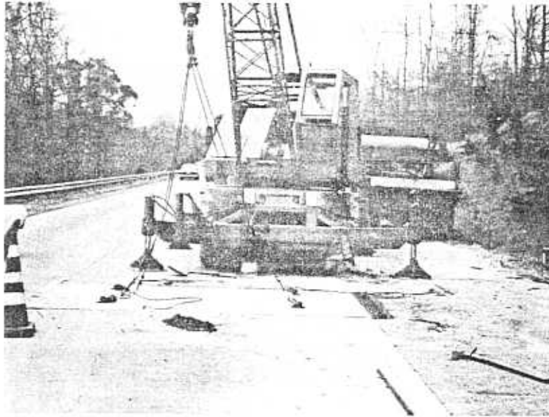
Figure 27. Precast slab in place.
