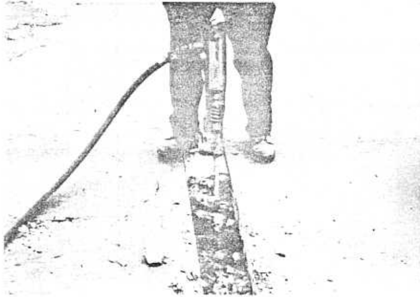
Figure 21. Stress relief at one end of repair area requiring third transverse sawcut (Michigan photo).
