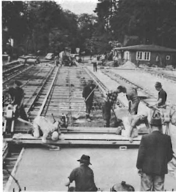
Figure 8: Concreting a strip of slab.
