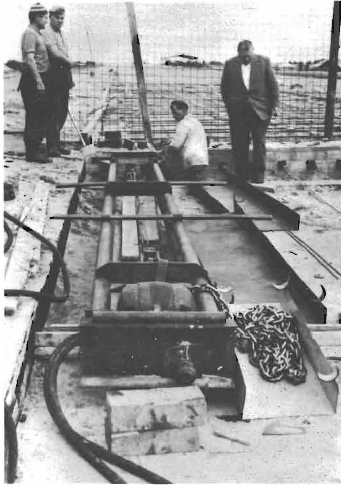
Figure 11: Jack for producing tendon extensions up to 4.50 m.
