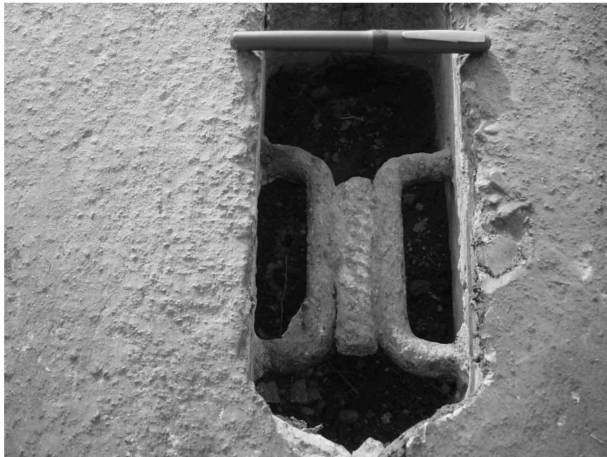
Figure 2. Example of PAG XIV precast airfield slabs (probably constructed early 1980s, still in service).
