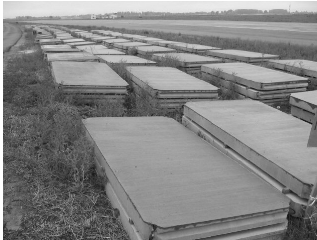
Figure 4. Precast slabs stockpiled at previous Soviet military airfield to be used for rapid runway repair. Note this is not one of the standard precast slab designs discussed in the paper.
