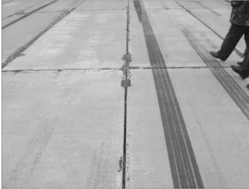
Figure 2. Example of PAG XIV precast airfield slabs (probably constructed early 1980s, still in service).
